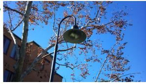
of fixtures, that way the Facilities Management crew can retrofit the energy wasting fixtures to more energy efficient ones. The retrofitting process will not require removing the entire fixture. This process only requires replacing the current lighting bulb in the cage to an energy efficient one. After the retrofit from a 200 watt to a 70- 100 watt fixture UC Irvine will be able to save money and at the same time save the environment, allowing UCI to become a greener school.
